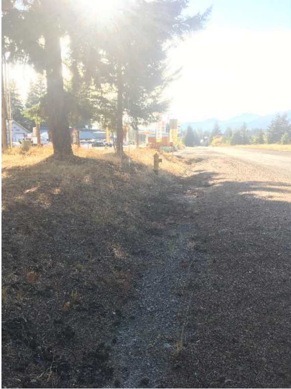
Figure 11: Feature M- Gravel Swale, looking southeast along Sparks Rd
