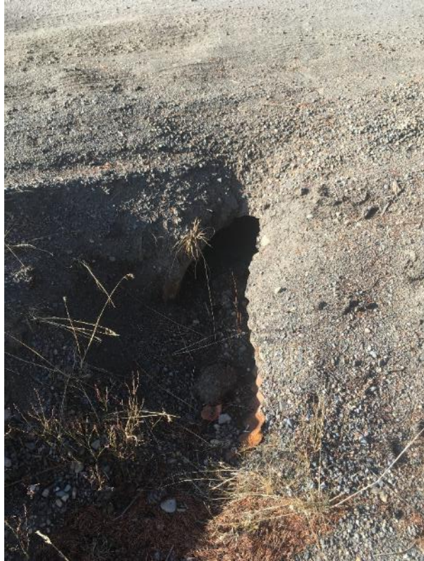
Figure 12: Feature O- 18" CMP entrance
