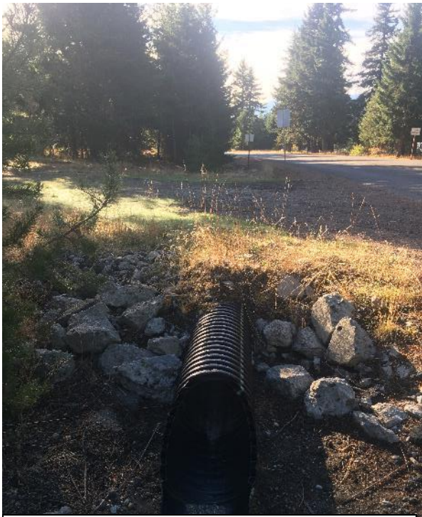
Figure 9: Feature J- 15" PVC culvert entrance
