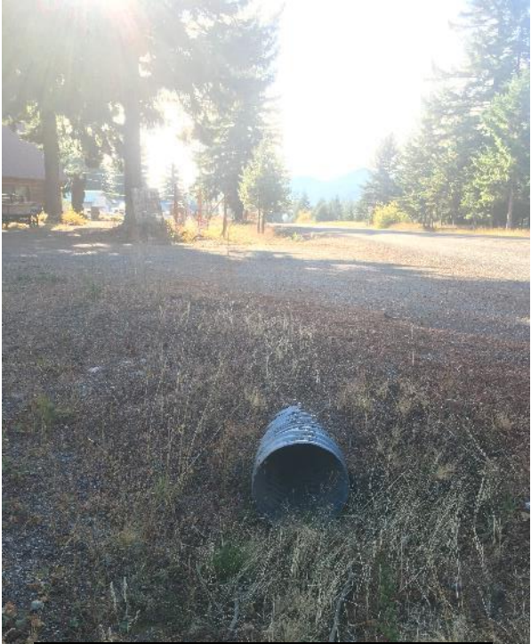
Figure 10: Feature L- 15" CMP entrance
