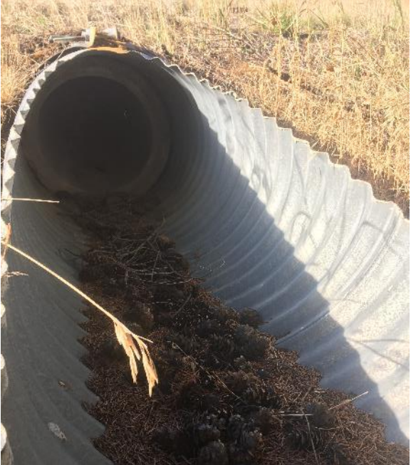
Figure 8: Feature I- 15" Concrete culvert entrance
