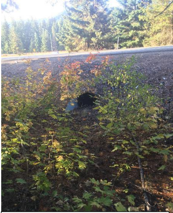
Figure 7: Feature H- 24" CMP entrance
